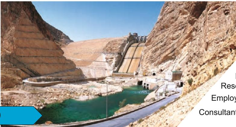
Dam Type: Rock-fill with clay core
