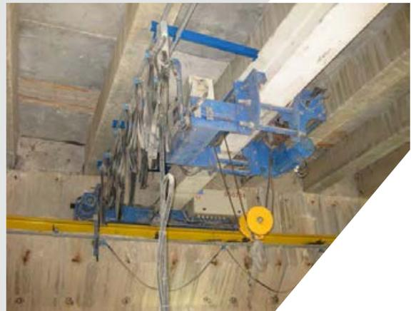
**Drilling equipment and cut off wall,
